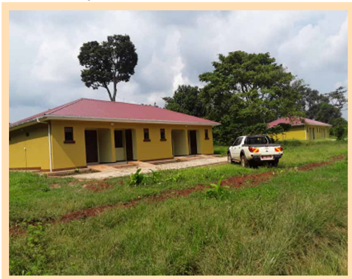
Figure 23: new residential units for staff at NaCORI
