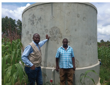
A concrete water tank reservoir of 30,000 litre-capacity at Kaahwa's farm
